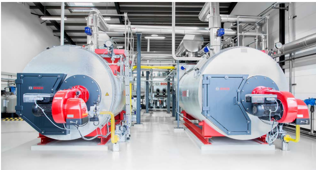
The two efficient Bosch steam boilers supply a total of up to 8 t/h of steam. 1,900 MWh a year. Furthermore, the minimised CO 2 emissions improve the ecological balance.
