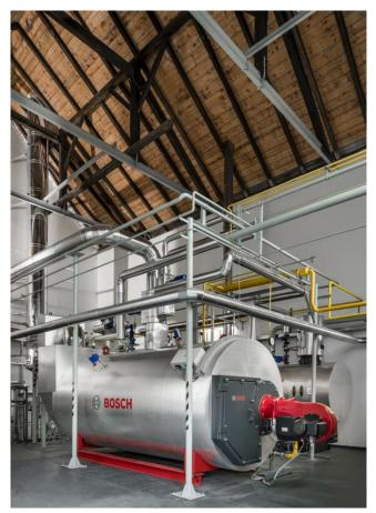
The steam boiler UL-S from Bosch efficiently supplies brewhouse, bottle and keg cleaning with steam.
