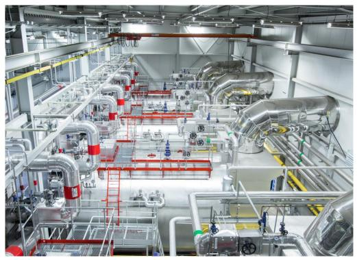
The boilers can produce up to 167 tons of superheated steam per hour for starting up the steam turbine and supporting the district heat supply.
