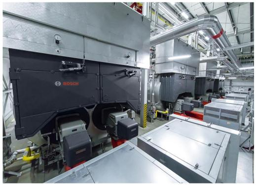
Each of the boilers are equipped with two natural gas burners, both single and parallel operation is possible.
