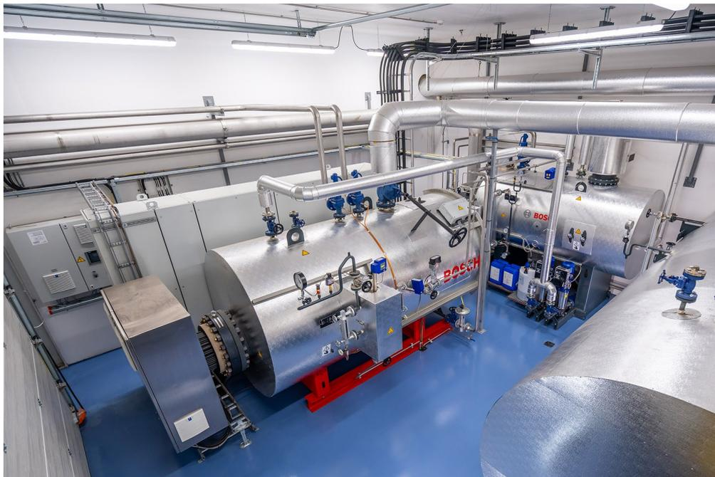
Image\_03: Electrical steam boiler system from Bosch with 100 per cent green energy utilisation.
