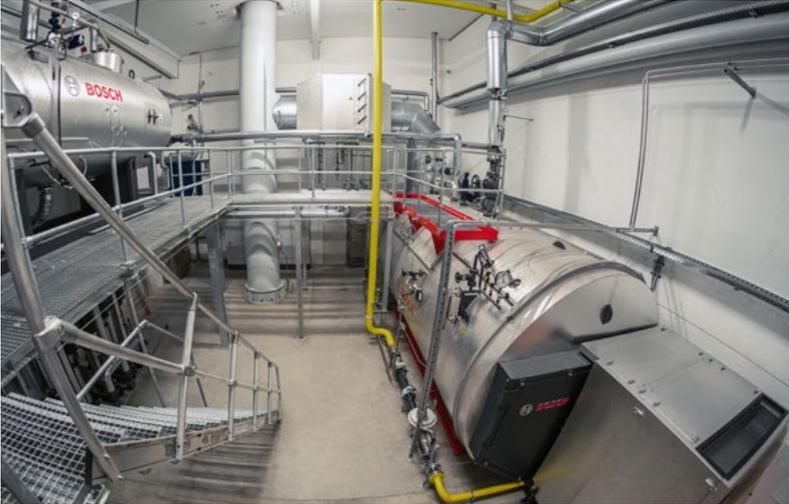
Figure 8: Hans Heinglein und Sohn GmbH's particularly efficient steam boiler system with an integrated economiser and downstream flue gas condenser.
