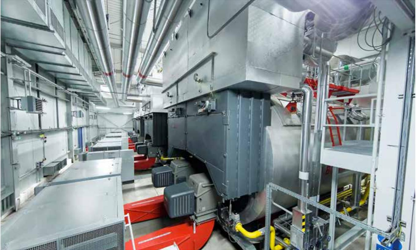
Figure: Four Double-Flue Boilers UNIVERSAL ZFR with superheater module
