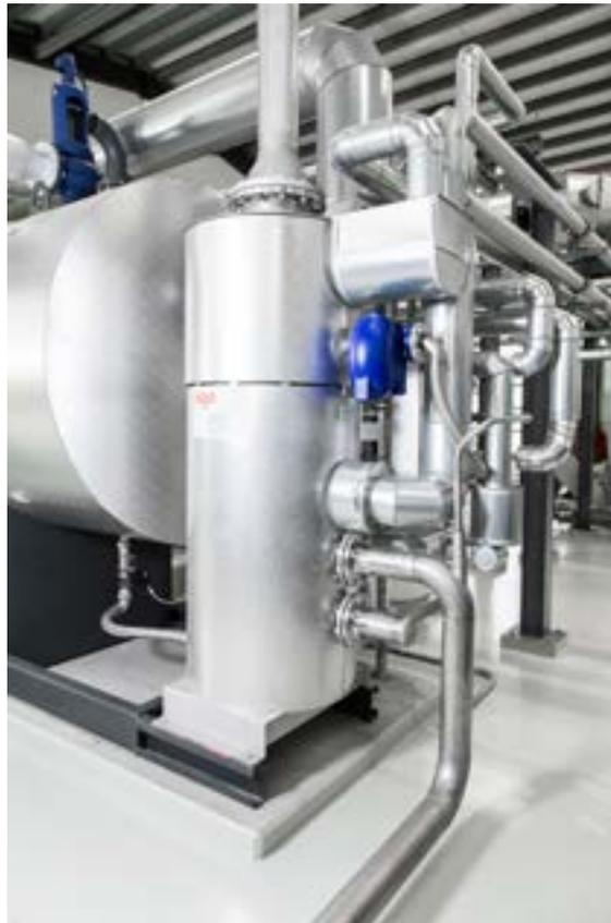
**Fig. 157** Expansion and heat recovery module EHB
