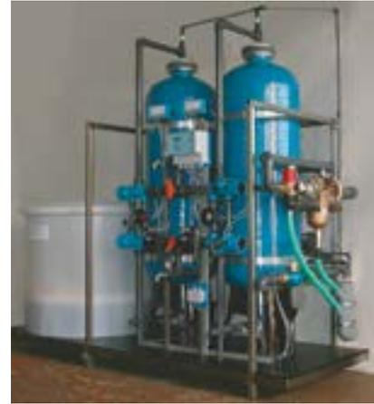
**Fig. 92** Schematic and visual representation of a dual water softener system
