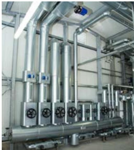
**Fig. 199** Steam distributor SD in existing system
