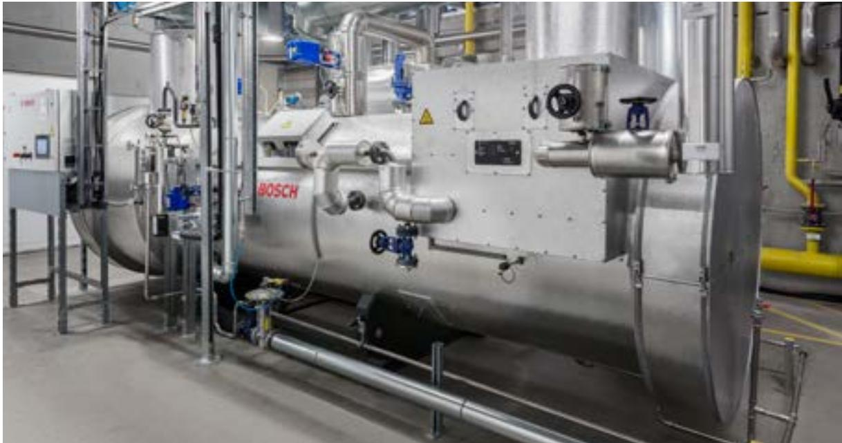
Fig. 191 UNIVERSAL heat recovery steam boiler HRSB system
