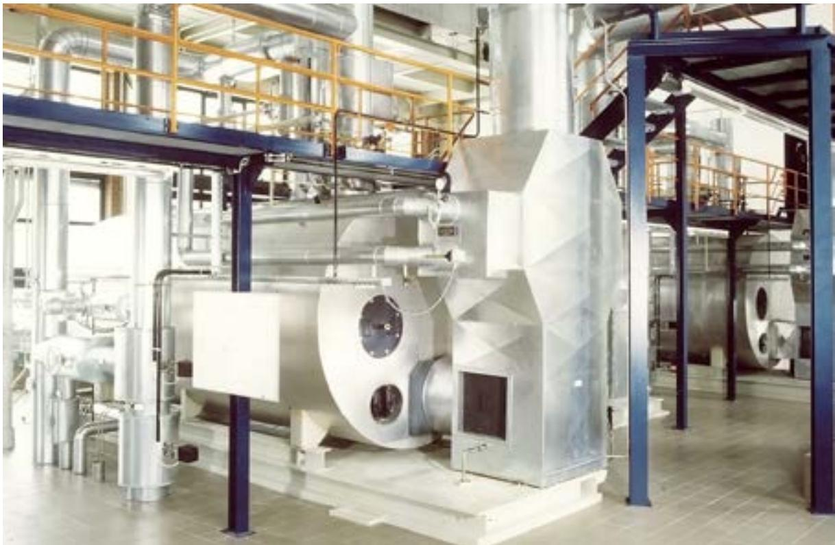
**Fig. 67** Standalone economiser in combination with a dual combustion system (gas/heavy fuel oil)
