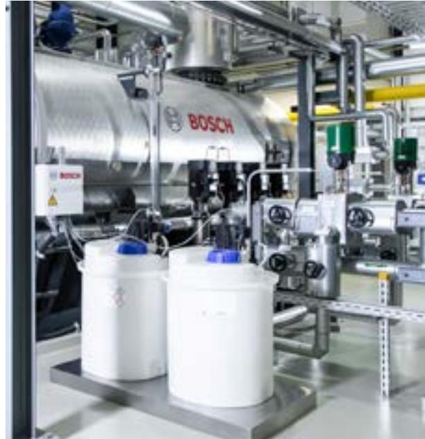
**Fig. 178** Water service module WSM
