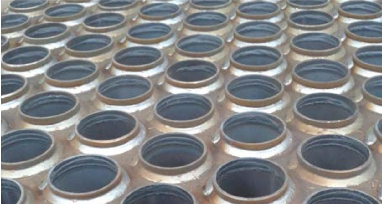
**Fig. 129** Weld seams at inserted smoke tubes
