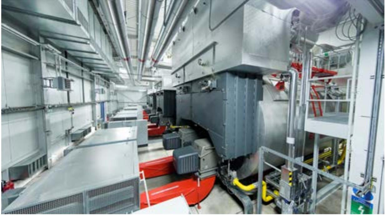
**Fig. 190** *Double flame-tube boiler with super heater module*
