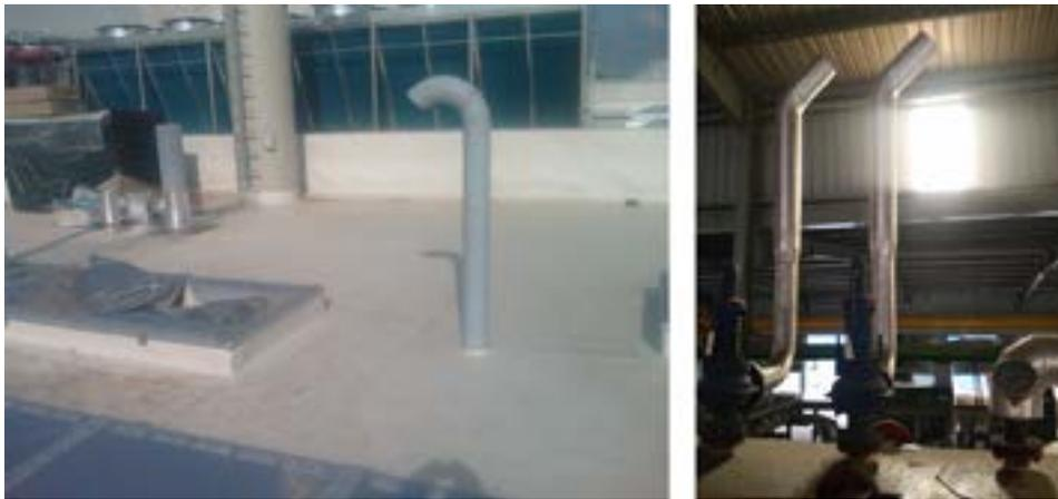
**Fig. 19** Safety valve blow-off pipe
