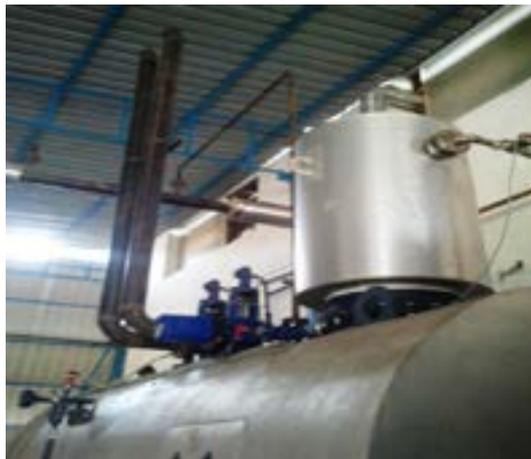
**Fig. 20** Holders of safety valve blow-off pipes missing
