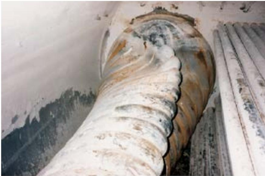
**Fig. 90** Layer formation in boiler with damage to flame tube
