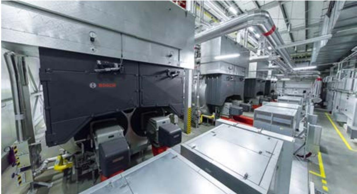
**Fig. 184** ZFR/ZFR-X steam boiler system
