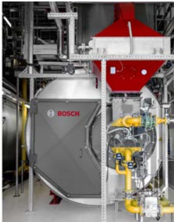
**Fig. 211** Air preheating system APH at a boiler
