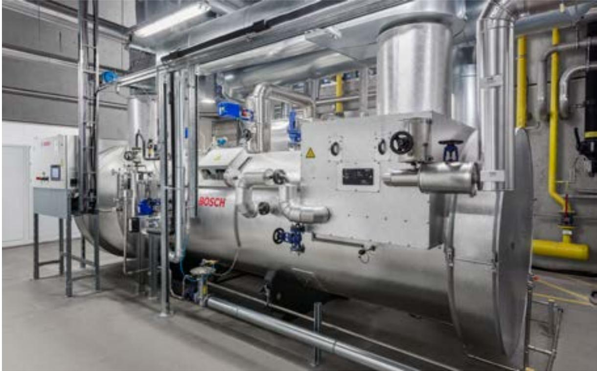
**Fig. 169** Bosch heat recovery boiler HRSB
