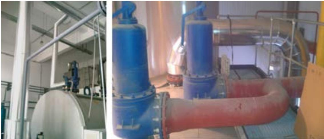
**Fig. 16** Impermissible merging of safety valve and expansion steam pipe
