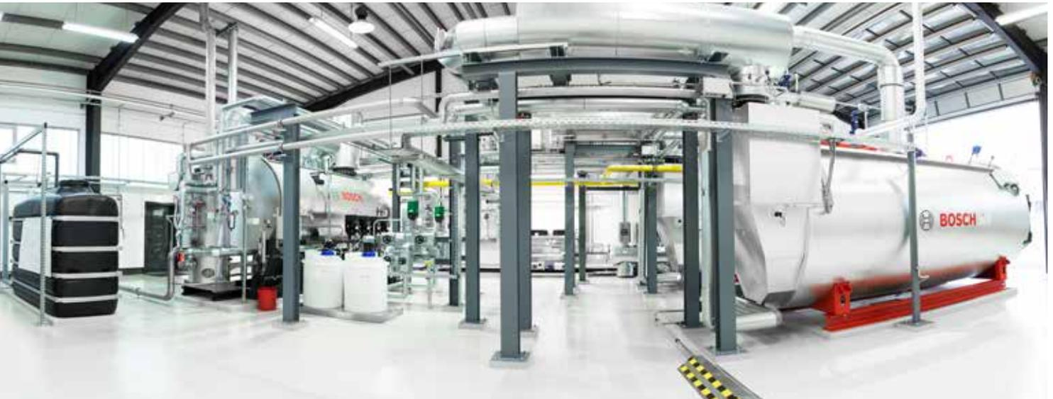
Water service module for deaeration (left) and the two UL-S steam boilers.
