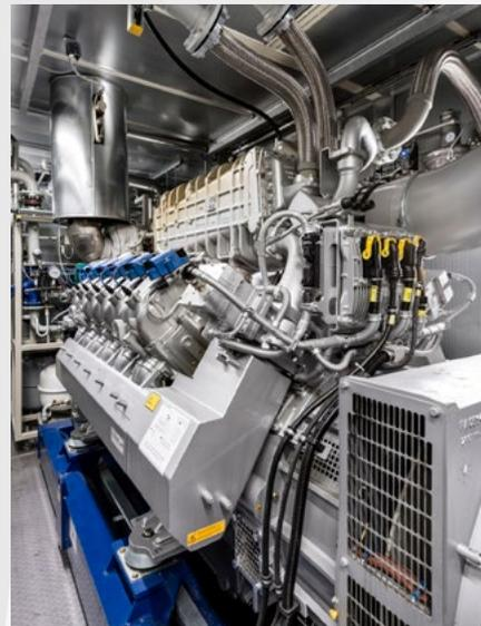
Highly efficient and resource-saving: The HRSB uses the waste heat from the CHP engine to generate steam.
