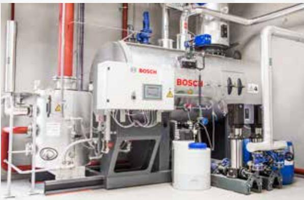
*The deaeration process of the feed water takes place within the water service module. By heating the water corrosive substances (carbon dioxide and oxygen) are removed.*
