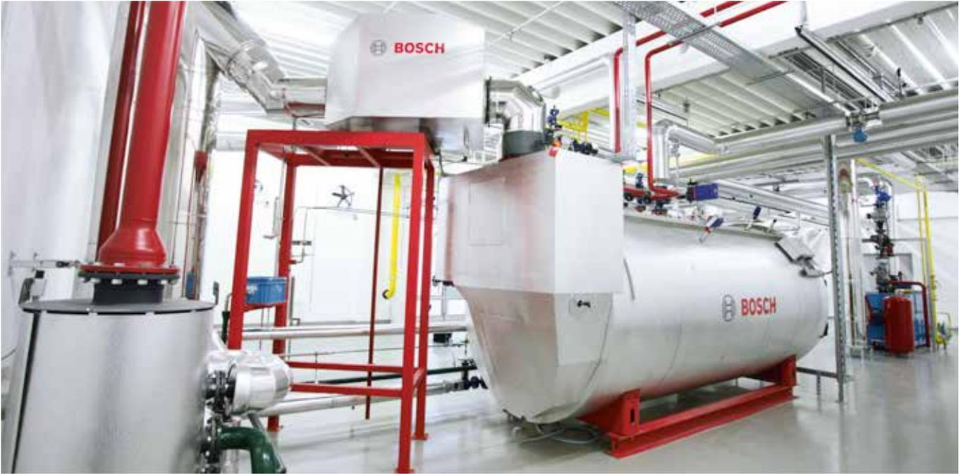
*Economizer and condensing heat exchanger for waste gas heat recovery.*
