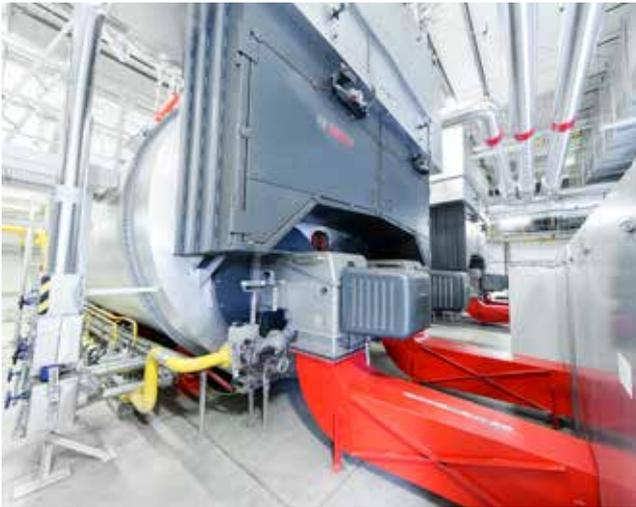
*Impressive power output: each of the eight burners has a combustion heat performance of 17.1 megawatts.*
