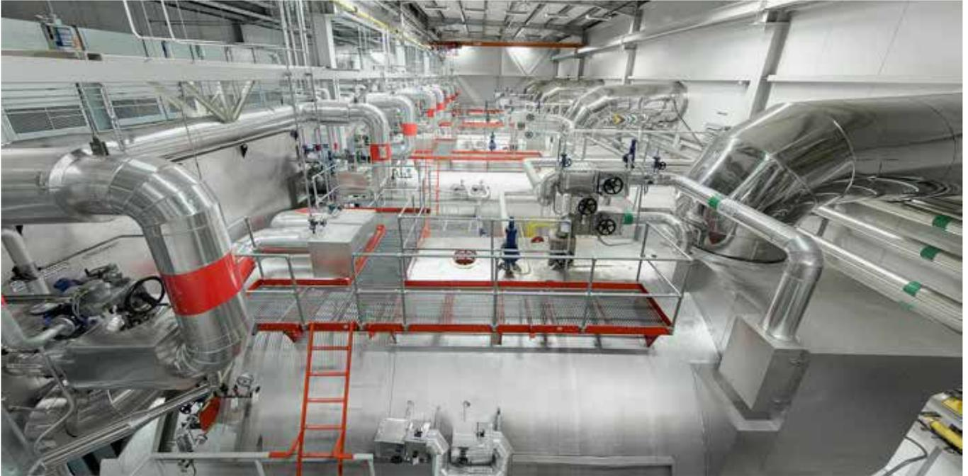
The four ZFR-X steam boilers each have an operating weight of 145 tons.
