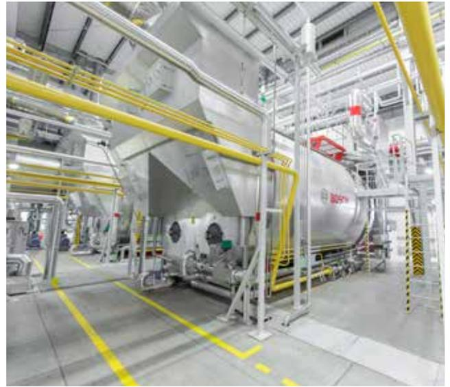
*High degree of efficiency: the economizers utilise flue gas heat to preheat the feed water thus saving large amounts of fuel.*
