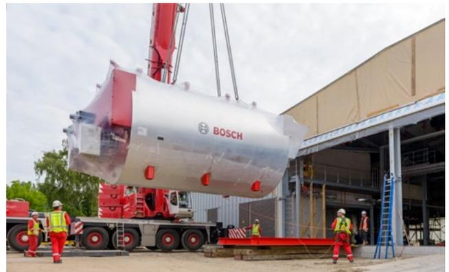
*Delivery and positioning – each boiler had a transportation weight of 68 tons.*
