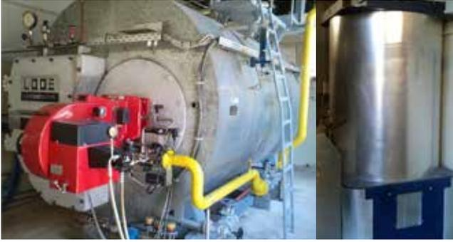
*Increased efficiency: The new firing with speed regulation and oxygen control as well as the retrofitted economizer.*
