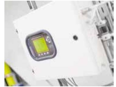
*O<sub>2</sub> and CO controls achieve optimum combustion.*
