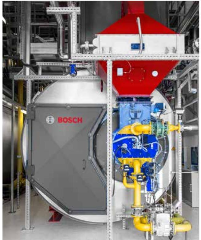
Energy-efficient Bosch steam boiler UL-S with air preheating system and twin-fuel firing system.
