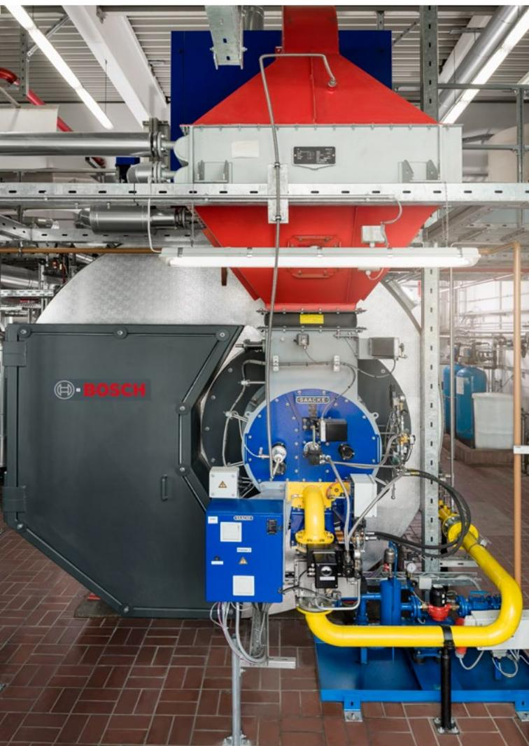
*The air preheating system reduces fuel consumption and emissions.*
