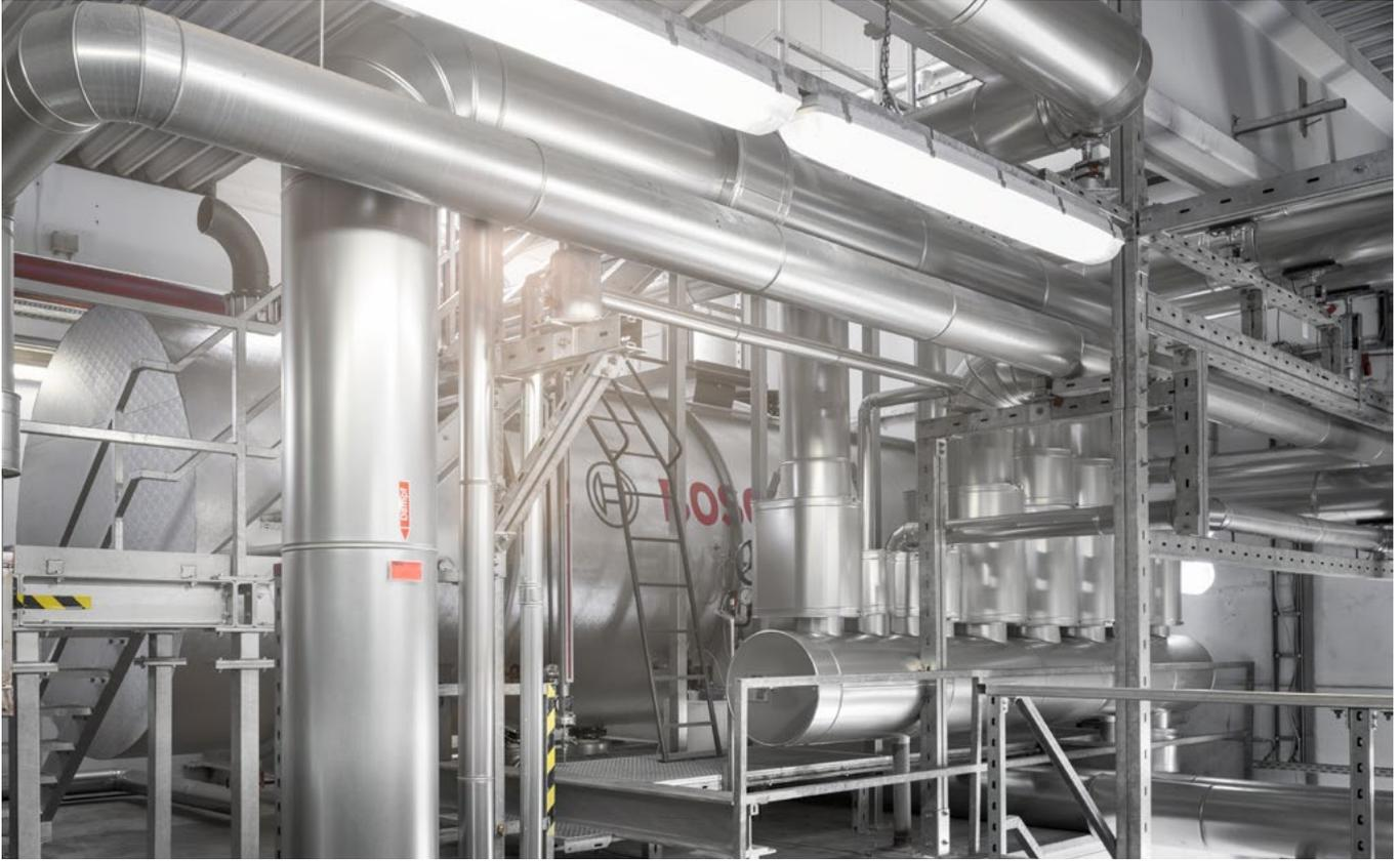
*The feed water deaeration module from Bosch provides optimum water quality and protects the boiler and components against corrosion. This increases the operational safety and the service life of the system.*
