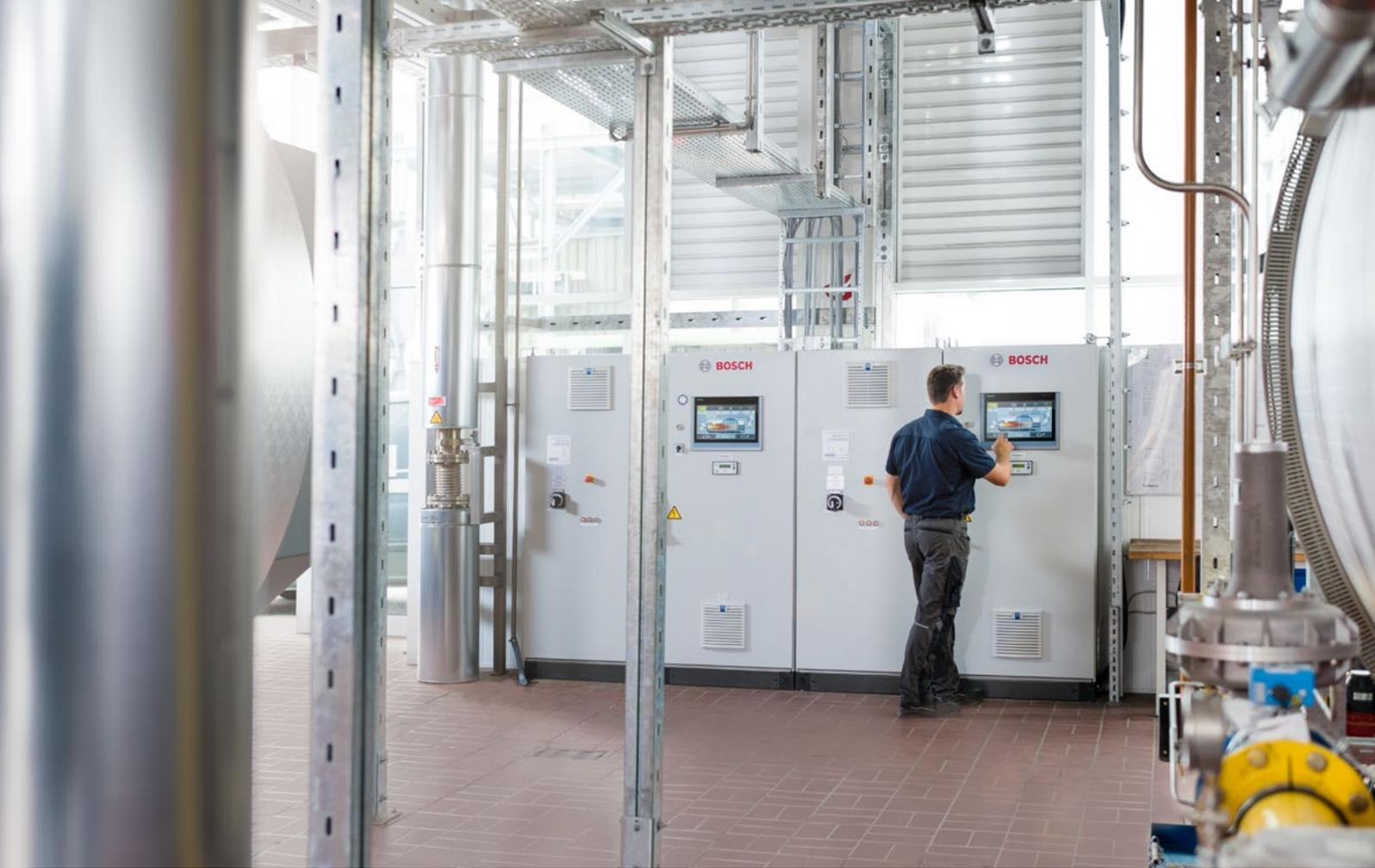
*The boiler controls ensure a high degree of automation and deliver relevant operating data to MEC Optimize.*
