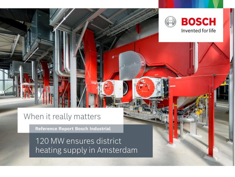
Four new low- $NO_x$  hot water boilers from Bosch have been connected to the district heating grid in Amsterdam in order to reliably handle consumption peaks and guarantee the supply as a round-the-clock backup solution.
