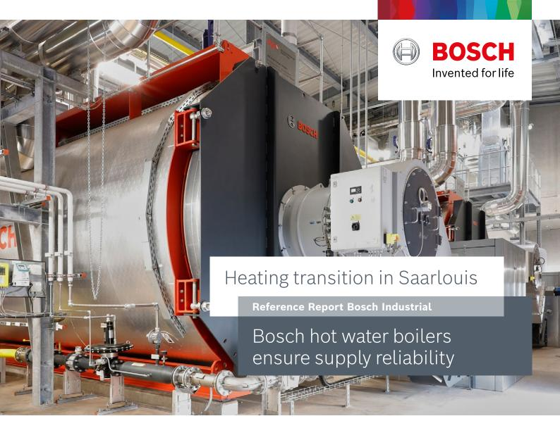
An important milestone in providing an eco-friendly supply of heat was reached by STEAG and Fernwärme-Verbund Saar (Saar district heating association). This included the use of two UT-M hot water boilers from Bosch, which act as a back-up and safeguard the supply at peak loads.
