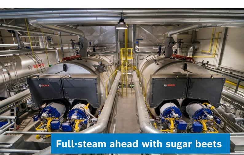
The system was ready right on time for the sugar beet campaign. In total, 72 tonnes of steam generated from two highly efficient Bosch double-flame tube boilers were put into operation at SLOVENSKÉ CUKROVARY s.r.o. in late summer of 2021. The project was impressive not only in terms of sustainability, but in many other ways.
