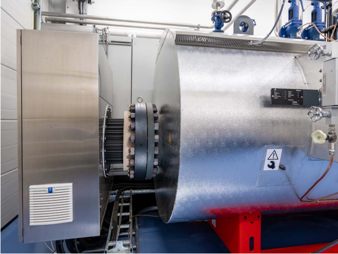
The stainless steel heating bundle is designed for a long service life
