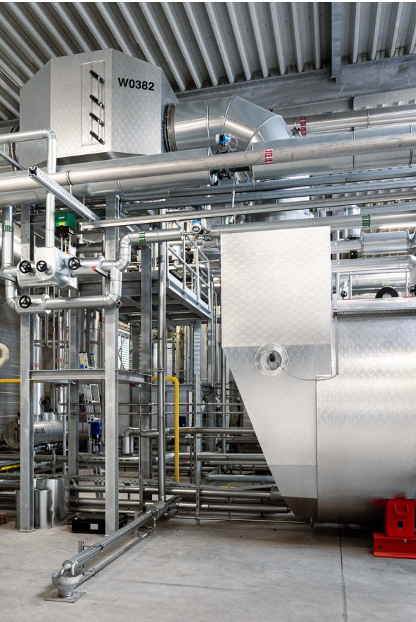
Economiser and condensing heat exchanger
