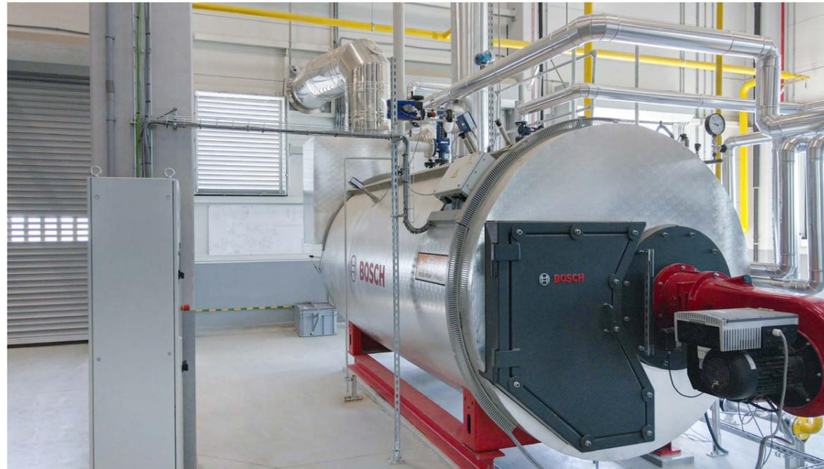
The UL-S steam boiler generates up to five tonnes of steam per hour and serves as a reliable back-up for the supply of steam.
