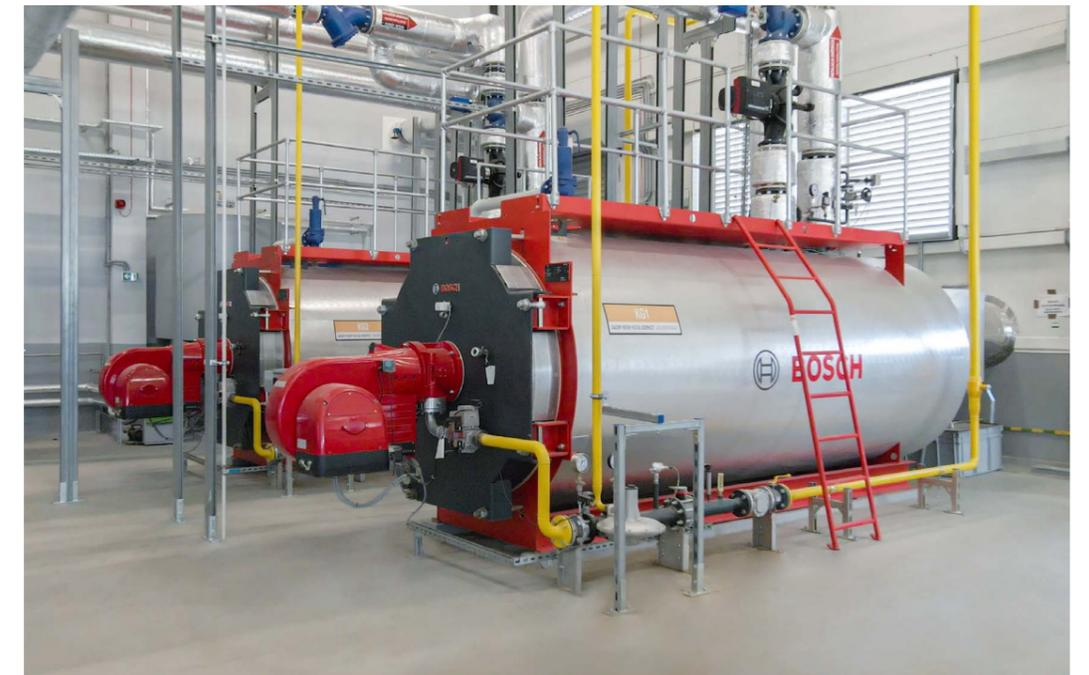
The Bosch UT-L boilers support the supply of heat to the buildings and are highly efficient in generating up to six megawatts of heat.
