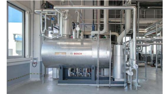
Bosch components, such as the thermal feed-water treatment system, complement the boiler system.
