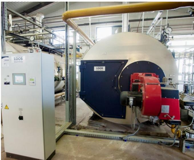
The steam boiler UL-S is used as back-up and for peak loads at Gallicoop.
