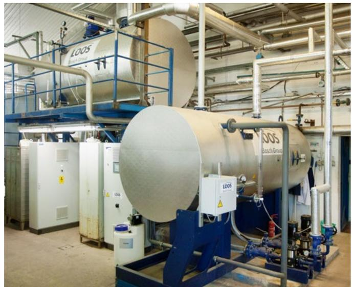
Deaeration plant (above) for corrosion-free feed water and condensate module for storage returning condensate.
