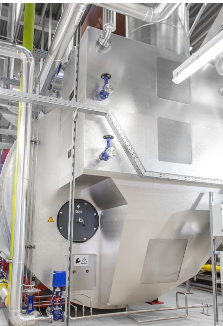
Figure 1: UL-S boiler with textured aluminium plate and insulated inspection openings
