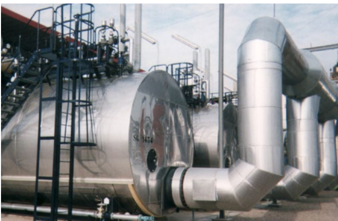
Figure 11: Weather-resistant insulation for the outdoor installation
