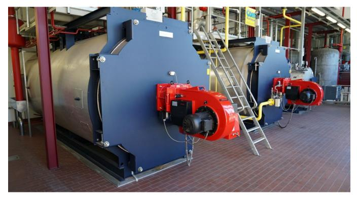
Two UNIMAT UT-H boilers generate a heat output of 7,000 kilowatts, and a UL-S UNIVERSAL steam boiler generates 1,250 kilograms of steam per hour.
