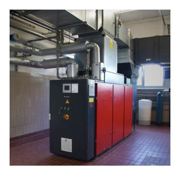
Operating for around 6,000 to 6,500 hours a year, the compressed air and heat system at Bahlsen covers the company's base-load need for compressed air.
