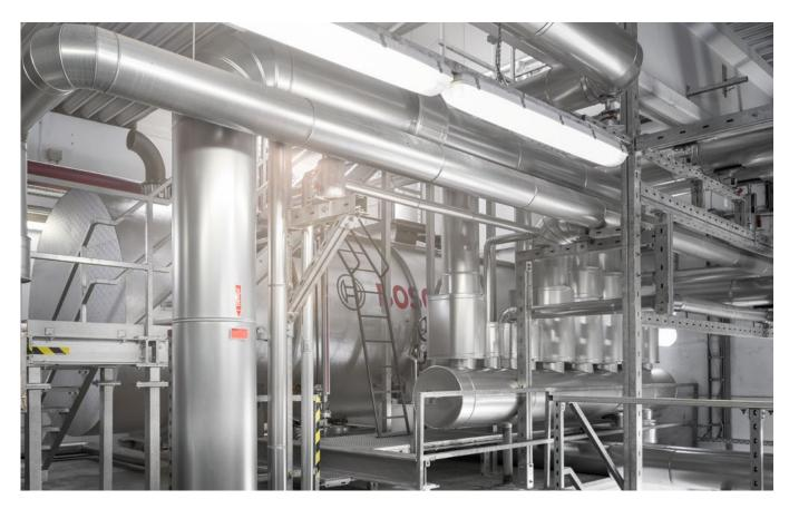
The feed water deaeration module from Bosch provides optimum water quality and protects the boiler and components against corrosion. This increases the operational safety and the service life of the system.
