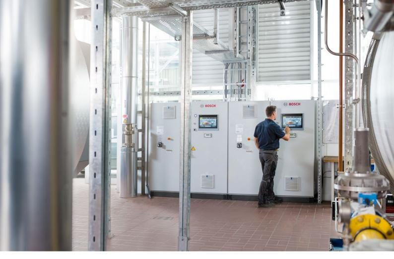
The boiler controls ensure a high degree of automation and deliver relevant operating data to MEC Optimize.
