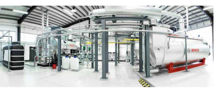
Water service module for deaeration (left) and the two UL-S steam boilers.
