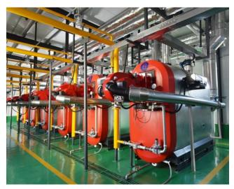
Part of the Uni Condens heating boiler systems from the first order in 2016 – each boiler generates 1.2 MW heat.
