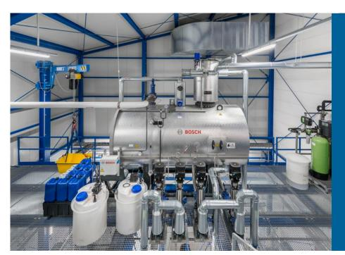
The WSM water service module is installed on the second level of the boiler house and provides the boilers with thermally treated feed water.
