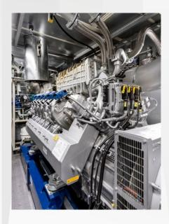
Highly efficient and resource-saving: The HRSB uses the waste heat from the CHP engine to generate steam.
