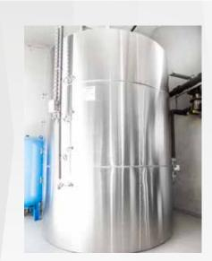
The solar thermal system supports the feed water heating with cost-free solar energy.
