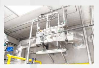
The condensation heat from the condensing heat exchanger (image) and the heat from the exhaust vapours heat up the make-up water prior the deaeration process.
