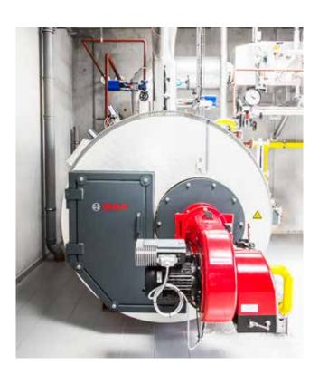
the number of times the burner is switched on and off, for example) are saved and displayed via the control systems. Further, they are equipped with integrated monitoring and protective functions to prevent incorrect operation. A remote service connection is also available, allowing the Bosch service engineers to access, analyse and optimise the operating data remotely.
