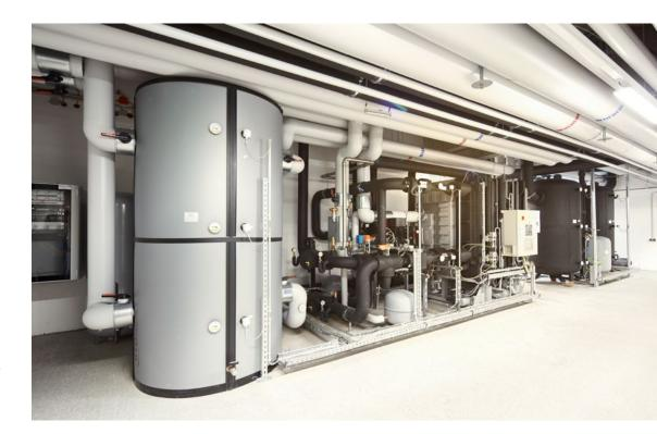
Whenever a lower heat requirement prevails, the connected absorption chiller generates 190 kW cold with the occuring waste heat of the CHA.
