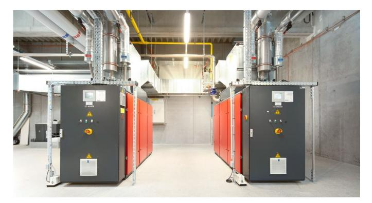
The two compressed air and heat systems from Bosch supply the company building with the base load requirement of compressed air of  $17.5 \text{ m}^3$ /min and 250 kW heat output.
