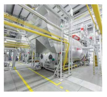
High degree of efficiency: the economizers utilise flue gas heat to preheat the feed water thus saving large amounts of fuel.
