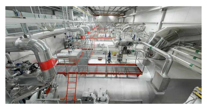
The four ZFR-X steam boilers each have an operating weight of 145 tons.
