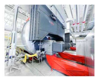
Impressive power output: each of the eight burners has a combustion heat performance of 17.1 megawatts.
