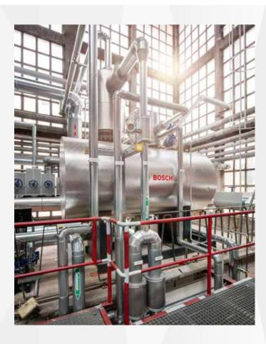
The feed water deaeration system was placed one floor higher in Pirmasens. Heating the feed water to 103 °C ensures that corrosive elements in the feed water dissolve. To make the process more efficient, a downstream vapour cooler uses accumulating exhaust vapour to pre-heat make-up water.
