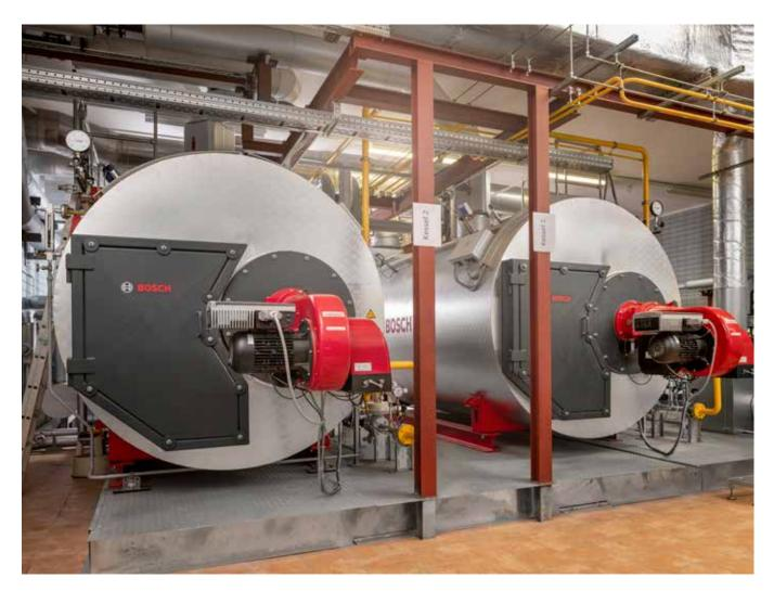
The Bosch boilers in Bellheim supply the brewery for processes like mashing and boiling. A cascade control ensures exceptionally cost-effective operation of the multi-boiler system.
