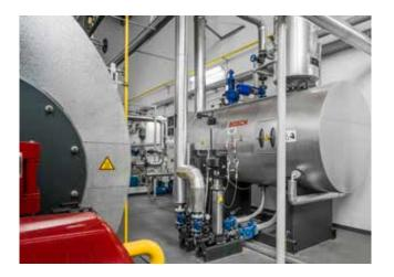
The deaeration module from Bosch protects boiler and components from corrosion and increases operating safety. The module is delivered pre-assembled from the factory and can be installed within shortest time.
