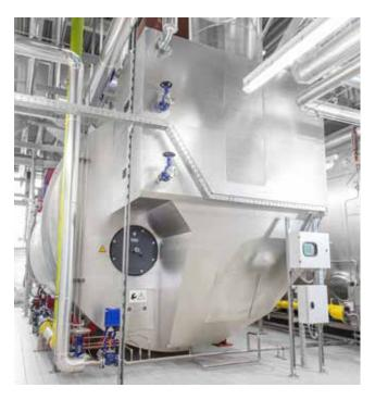
Effective use of waste heat with integrated economizer and flue gas heat exchanger.
