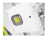
$O_2$  and CO controls achieve optimum combustion.
