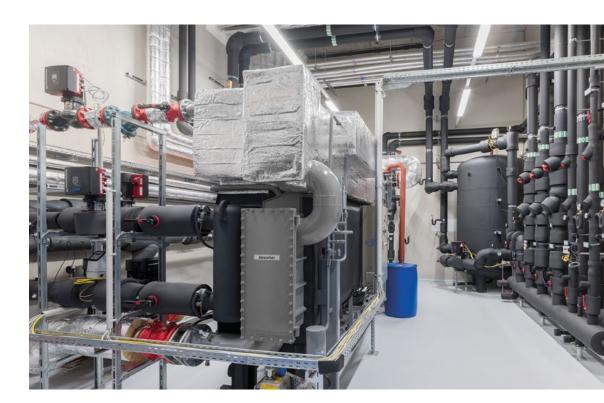
Whenever there is a reduced heat demand, the connected absorption cooling machine generates cold to cool the site.
