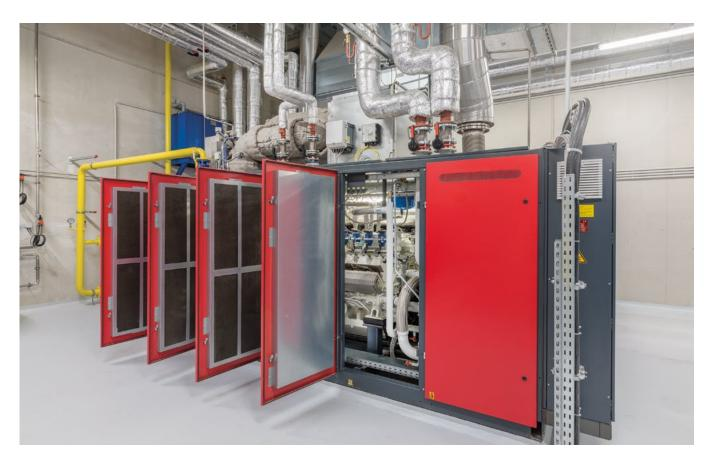
The Bosch CHP system supplies the site with 400 kW of electrical and 500 kW of thermal output for power, heating and cooling.
