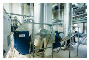
The waste heat boilers use the CHP waste heat for costefficient steam generation.
