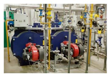
The two compact heating boilers UT-L produce the heat for operation of the fermenter.
