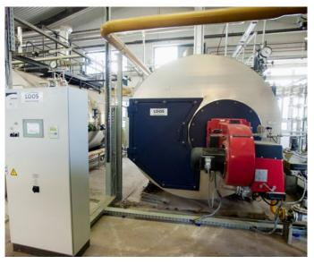
The steam boiler UL-S is used as back-up and for peak loads at Gallicoop.
