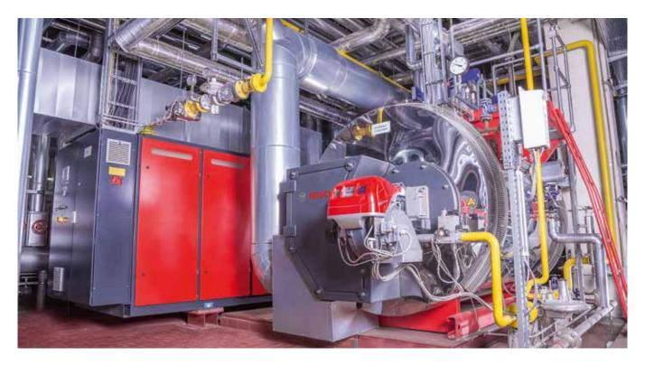
Effective use of waste heat sources: The CHP waste heat with temperatures of up to 550 °C are passed through the fourth pass of the steam boiler and used for the steam generation.
