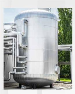
The waste heat from the compressors and cold stores is buffered in the heat storage tank.
