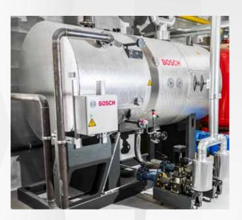
Reduction in make-up water quantities through use of condensate service module.
