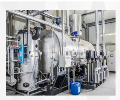
The water service module with heat recovery from the desalting water.
