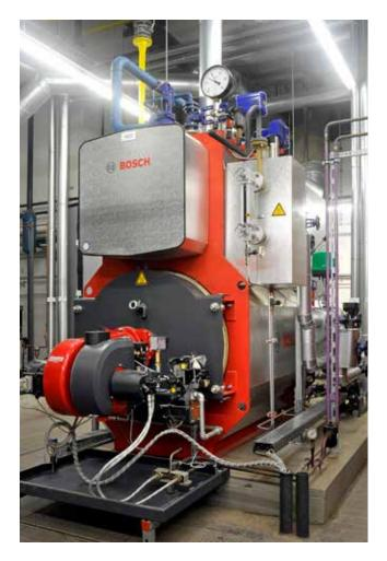
The compact steam boiler U-MB with an economizer and natural gas firing.
