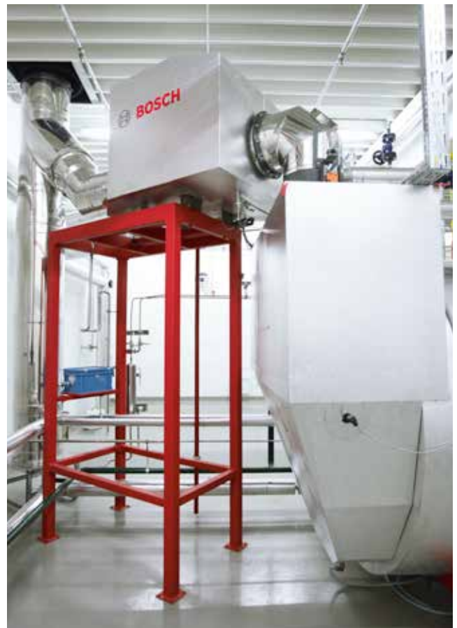
Integrated flue gas heat exchanger and flue gas heat exchanger for condensing use
