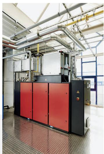
Image: Combined heat, power and compressed air system at the power station of the Bosch Thermotechnik GmbH in Lollar
