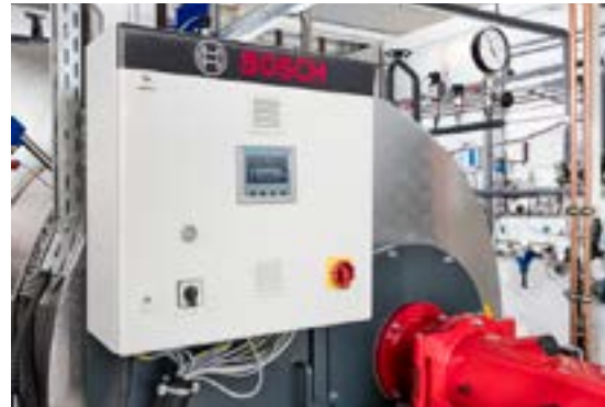
Fig. 174 Compact steam control CSC for the steam boiler CSB
