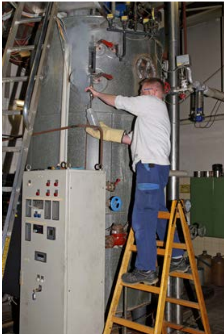
Fig. 34 Water sampling without suitable cooler and with unsuitable container
