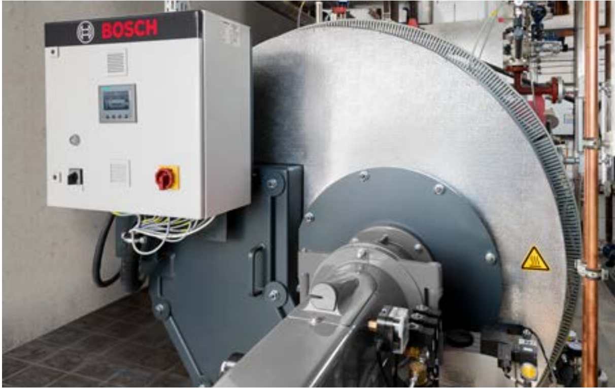
Fig. 85 Compact control cabinet of CSC for steam boilers in the smaller output range
