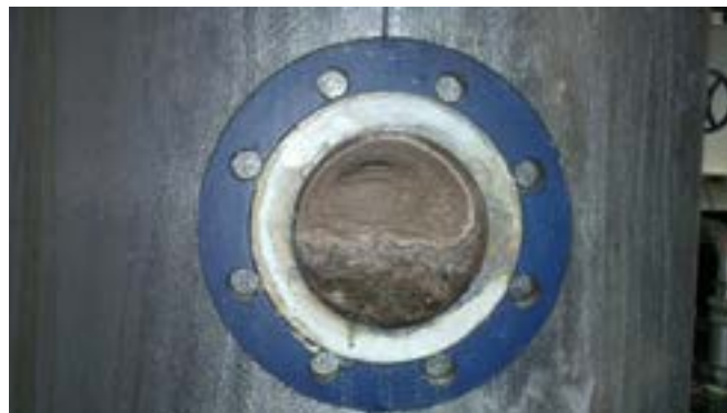
Fig. 32 Overflow at BEM removed; complete calcification at BEM
