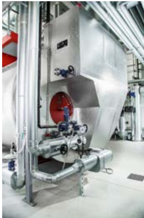
Fig. 62 Heat maintenance coil installed in base of boiler
