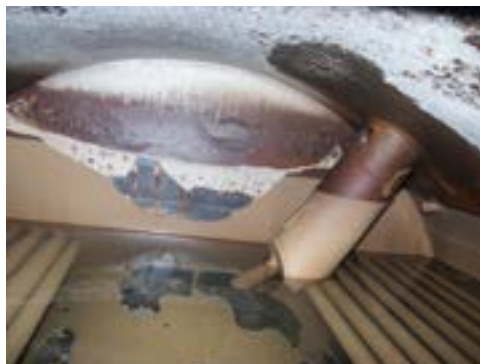
Fig. 23 Water-side deposits on the tube panel and tube plate of the boiler
