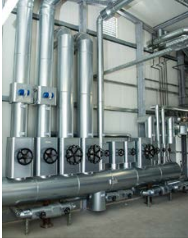
Fig. 182 Steam distributor SD
