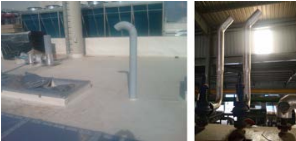
Fig. 19 Safety valve blow-off pipe
