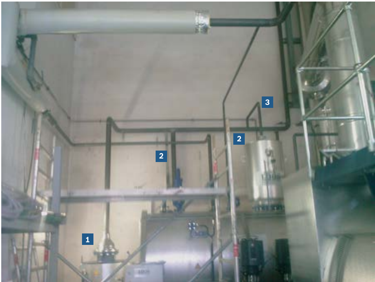
Fig. 18 Tapering (1) of expansion steam pipe on the bottom blowdown vessel. Merging (2) of expansion steam pipe, safety valve blow-off pipe and exhaust vapour pipe. Exhaust vapour pipe not made of stainless steel (3).
