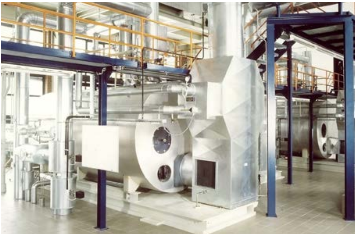
Fig. 67 Standalone economiser in combination with a dual combustion system (gas/heavy fuel oil)
