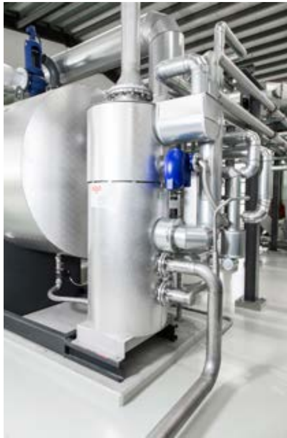
Fig. 157 Expansion and heat recovery module EHB
