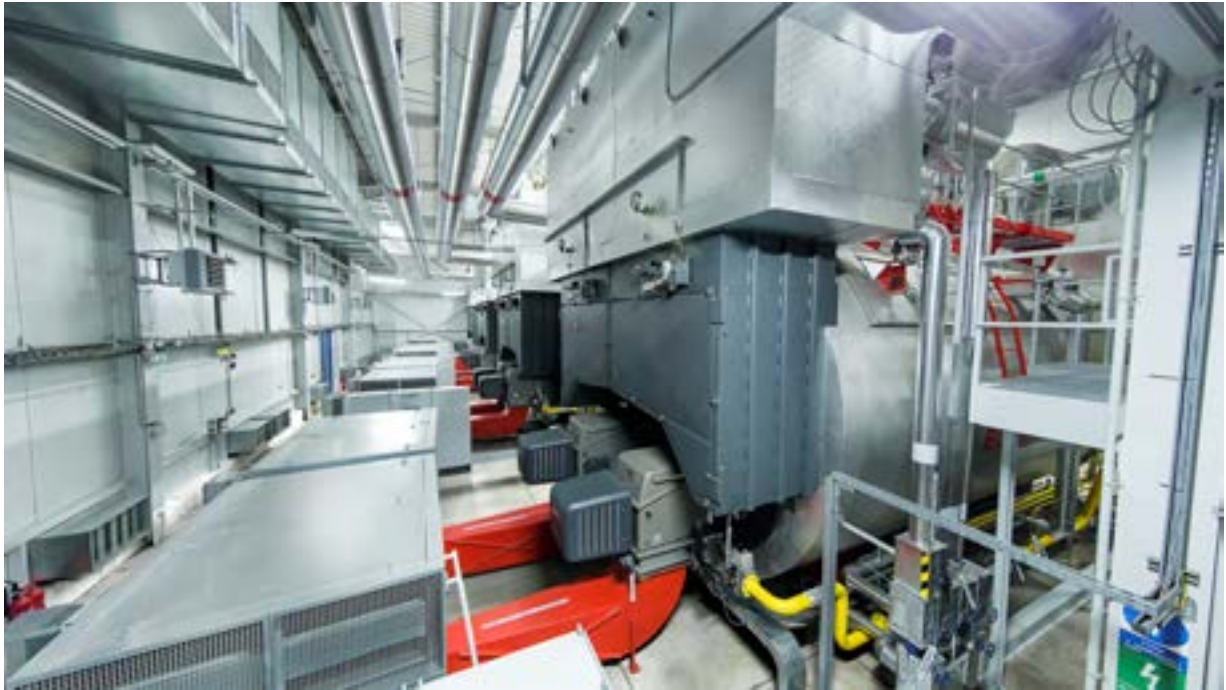
Fig. 190 Double flame-tube boiler with super heater module
