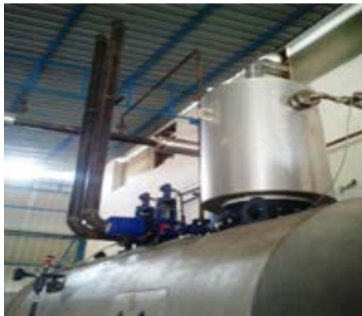
Fig. 20 Holders of safety valve blow-off pipes missing
