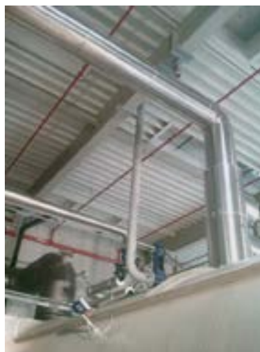
Fig. 21 Thermal expansion of safety valve blow-off pipes not possible
