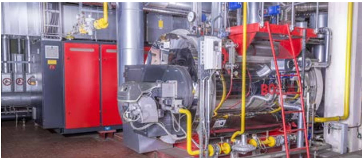
Fig. 61 Combined heat and power unit with 4-pass waste heat boiler
