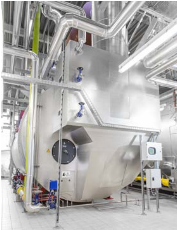
Fig. 165 Removable insulation at inspection apertures (UL-S with integrated economiser)
