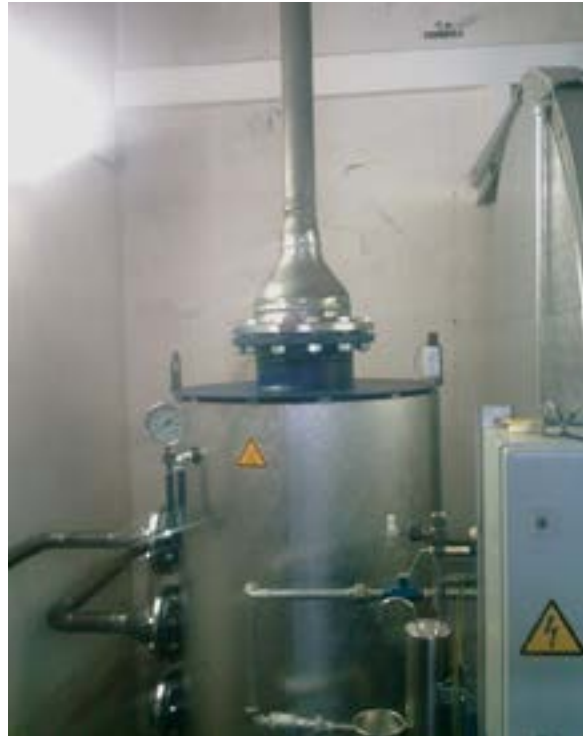
Fig. 17 If the internal diameter of expansion steam pipes is reduced, this can lead to an increase in pressure and rupturing of the vessel
