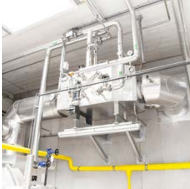
Fig. 186 Flue gas heat exchanger ECO 6 for condensing use
