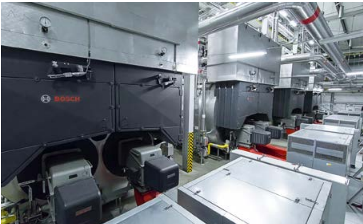
Fig. 73 Double flame-tube boiler with mounted superheater on top
