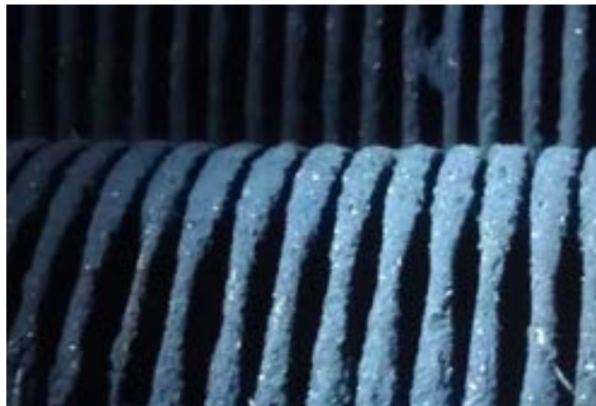
Fig. 29 Deposits on the ribs of the economiser
