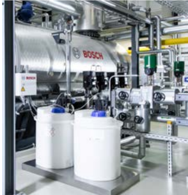
Fig. 178 Water service module WSM
