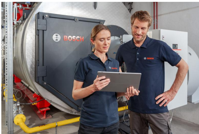
Image_02: Expert on-site consultation: Optimised processes, lower energy consumption and CO 2 emissions, and enhanced operational reliability.
