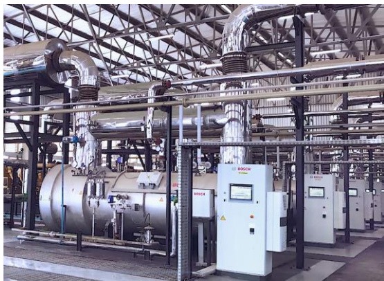
The heat recovery steam boilers from Bosch generate 20 percent of the steam demand at International Breweries Plc. using waste heat.
