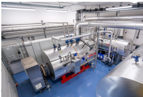
Electrical steam boiler system from Bosch with 100 percent green energy utilisation.
