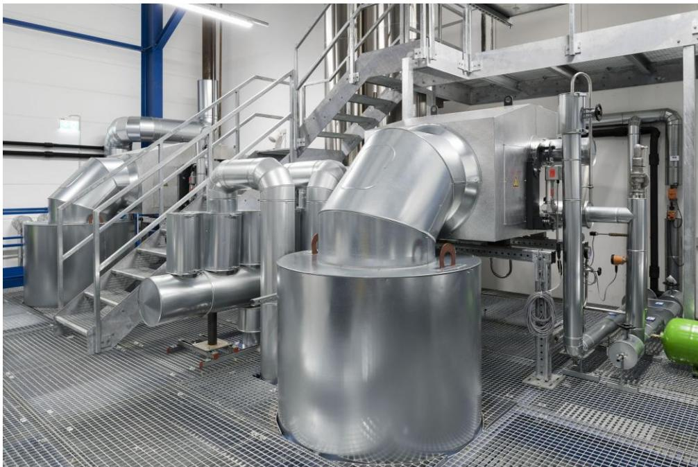
Residual flue gas heat from steam generation is used with condensing heat exchangers, and this means that fuel is saved.
