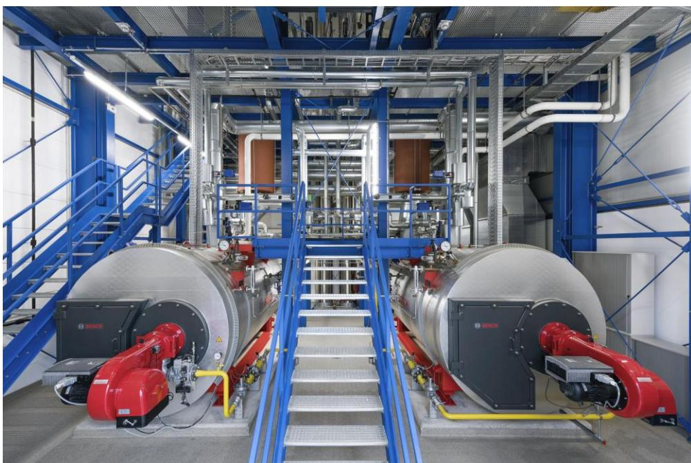
The two Bosch steam boilers deliver a total of up to 10,000 kilograms of steam per hour for manufacturing herbal medicines.
