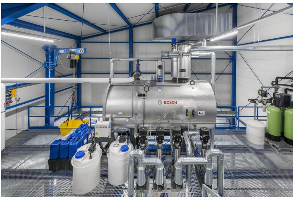
The WSM water service module is installed on the second level of the boiler house and provides the boilers with thermally treated feed water.
