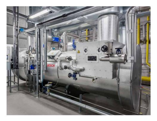
High-efficiency and resource-saving: The HRSB uses the waste heat from the CHP engine to generate steam.
