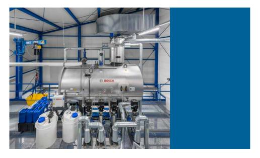
The water service module (WSM) is installed on the second level in the boiler house and provides the boilers with thermally-treated feed water.
