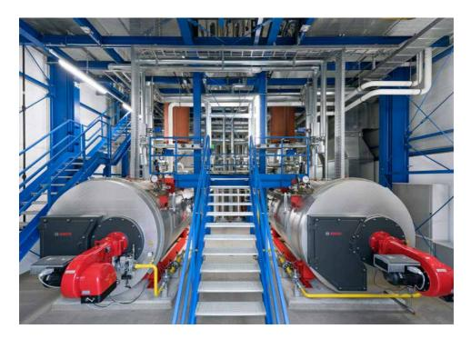
Impressive boiler house at Bionorica: The new boilers were sited on the ground floor. They deliver up to 10 t/h of steam in a highly-efficient and low-emission way.
