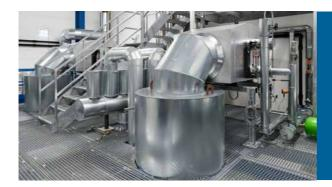
The condensing heat exchangers use the remaining flue gas heat from steam generation to heat up the water used in production.
