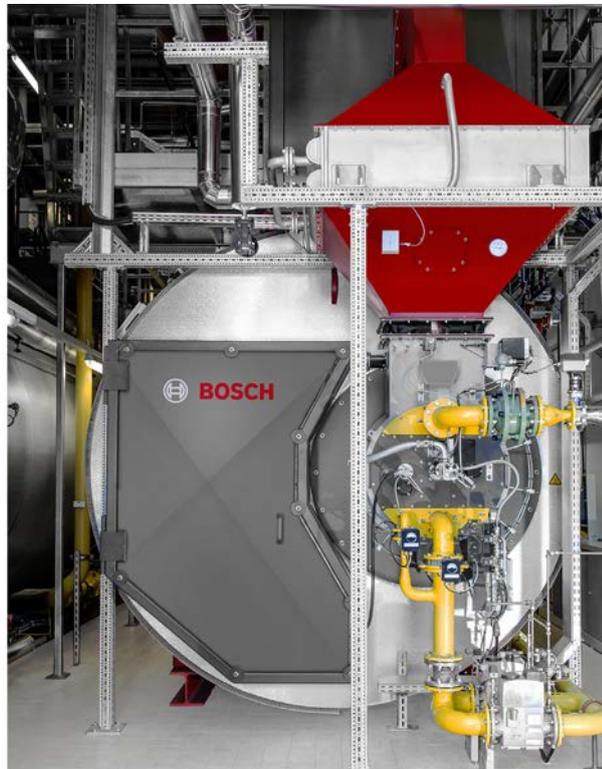
**Fig. 210** Air preheating system APH at a boiler
