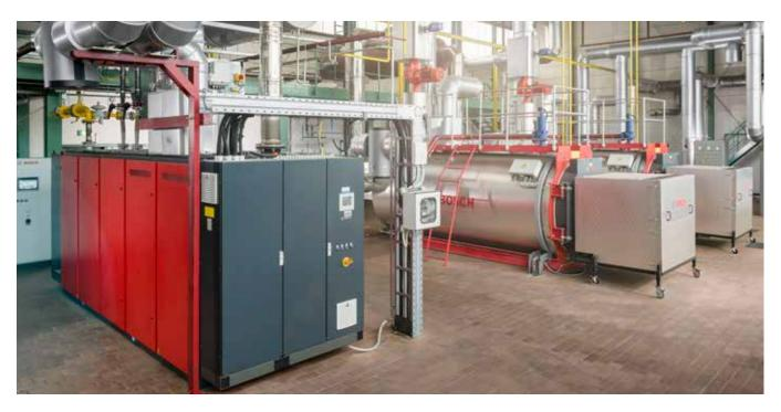
The Bosch CHP provides the base load for heating and at the same time electric power for the company's own consumption.
