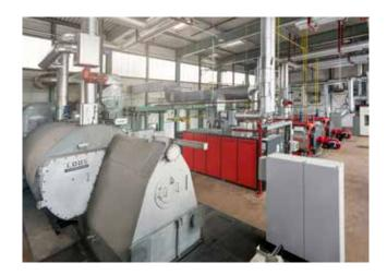
In operation since decades: The modernized Loos solid fuel boiler supports the heating supply.
